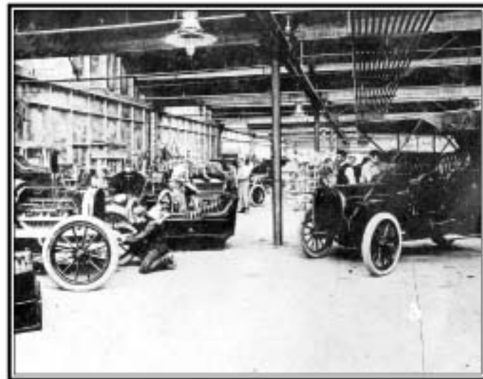
The Production Line
